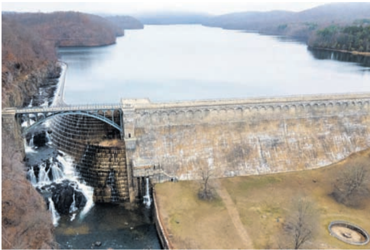
The New Croton Dam and the New Croton Reservoir that supplies part of New York City's drinking water is seen in Cortlandt, N.Y., on Thursday, March 20, 2025.
