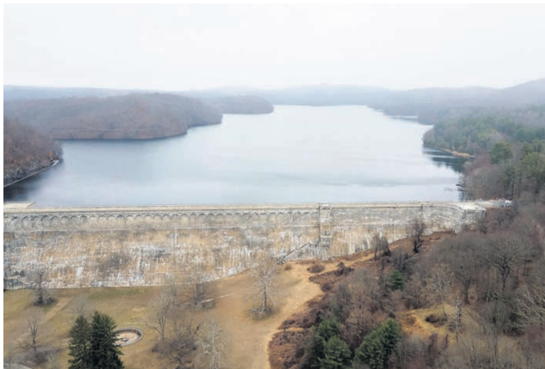
The New Croton Dam and the New Croton Reservoir that supplies part of New York City's drinking water is seen in Cortlandt, N.Y., on Thursday, March 20, 2025.
